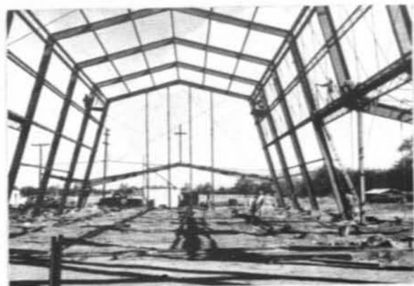
Church under construction, 1959
